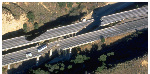
Northridge earthquake damage (Photo: FEMA)
