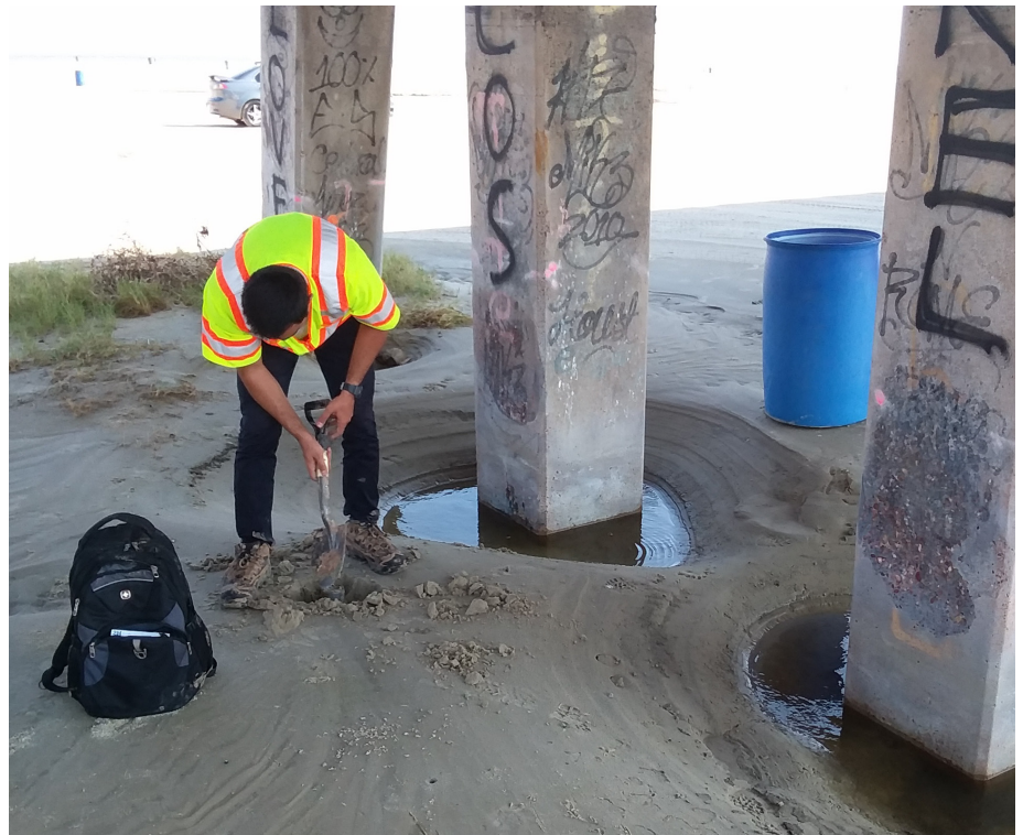
Infilled scour holes at the San Luis Pass. (Photo: Stephanie Smallegan)
