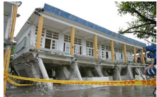
In-situ pushover test to verify the proposed technology for seismic evaluation and retrofit of school buildings
